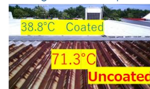
Coating on a folded plate roof
