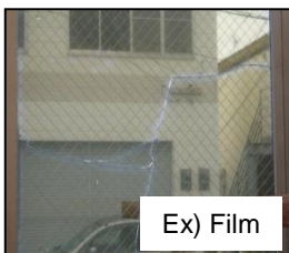
②heating crack
